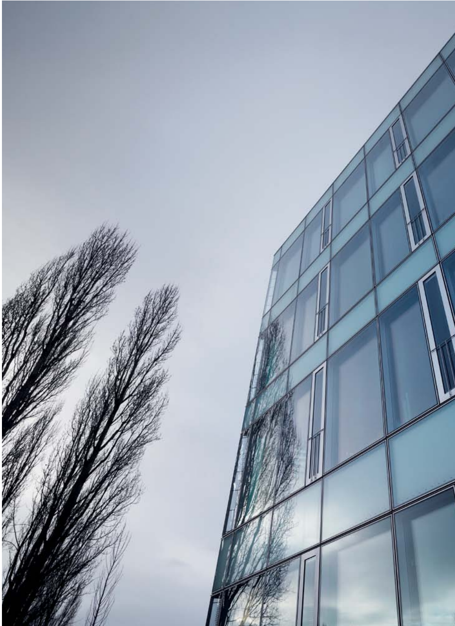
Triple glazing on the building's south face guarantees a high level of insulation
